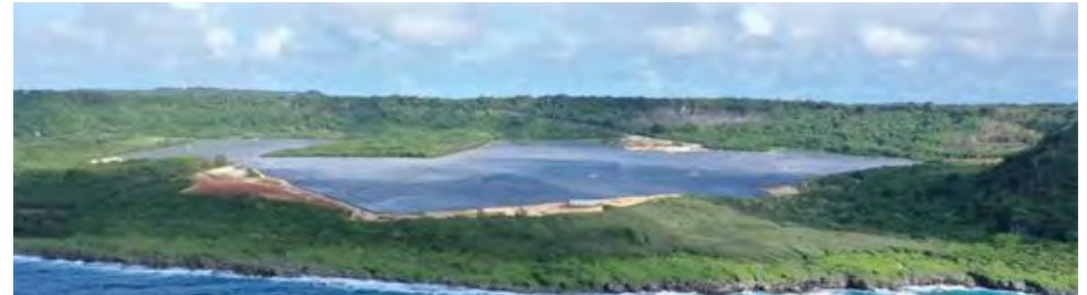
Renewable & Solar Assets
