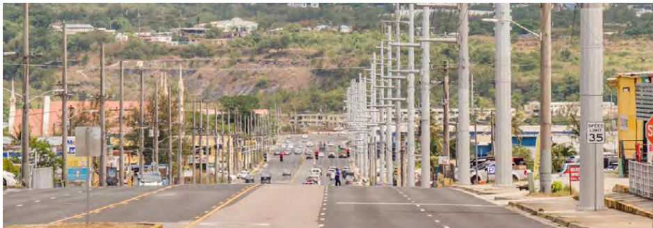
Hardened T&D — 170 mph rated poles
